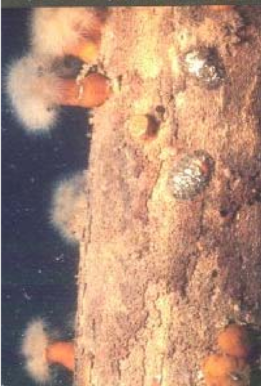
Plate 10. Marine borer attack ( Limnoria sp. ) on the untreated Mechanical Control piling recorded in October 1999, four years following construction.
