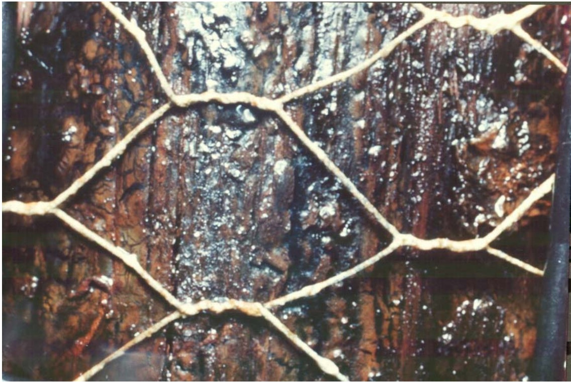
Plate 3. Close up view of the BMP piling surface taken at +10' Chart Datum showing the effects of solar heating four years after construction – October 1999.
